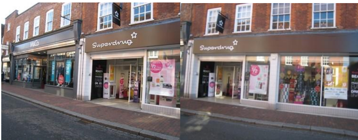
The shop on the left has divided the frontage with wooden painted windows and risers which fits with the street scene
