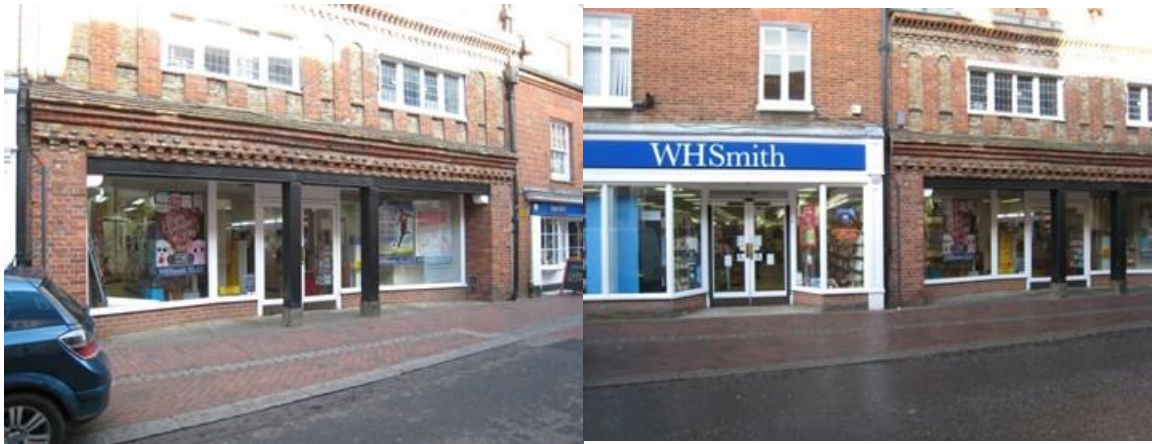
An example where the building's original features have not been spoilt by the shop front
