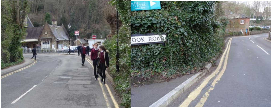
Lack of pavement on the station side of the main route into Godalming Town Centre
