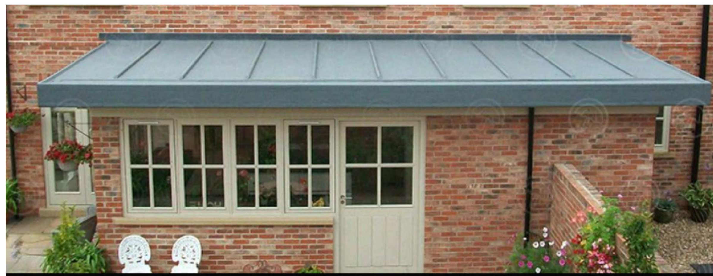
PRECEDENT TOPSEAL LIQUID ROOFING scale NTS
