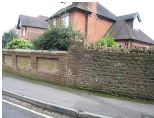
Original style Victorian brick and stone walls
