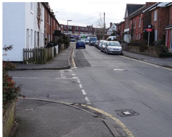
No dropped kerb at crossing, The Oval/Summers Road
