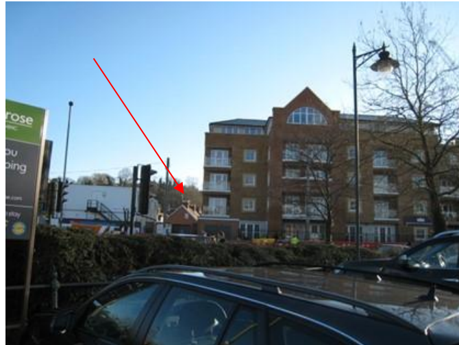
Flambard Way: Victorian terrace just visible (arrowed) to the left of Prime Place, but the hillside behind is no longer visible
