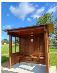
Replacement bus shelter in Eashing Lane
