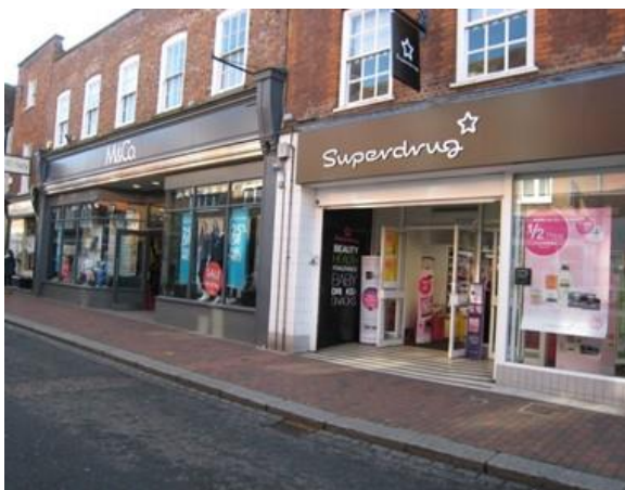
The shop on the left has divided the frontage with wooden painted windows and risers which fits with the street scene
