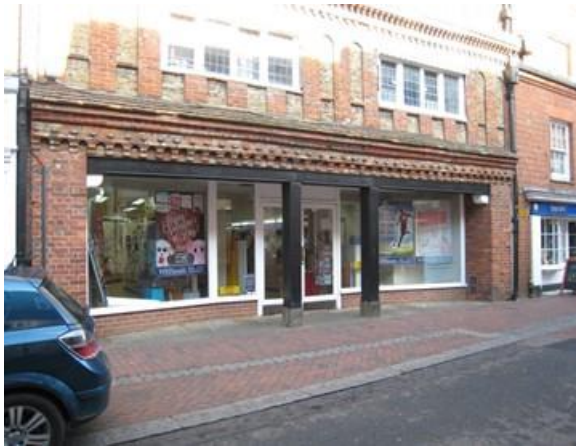
An example where the building's original features have not been spoilt by the shop front
