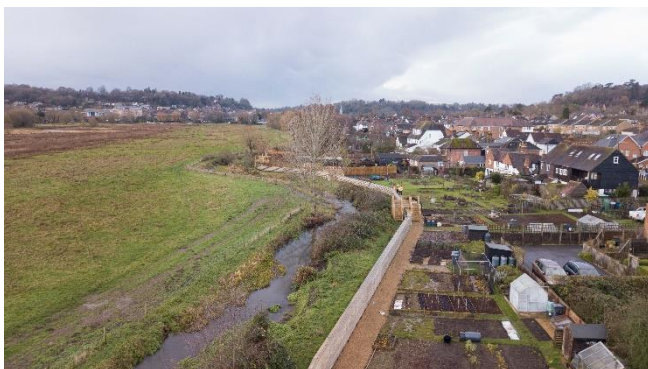
Aerial view of completed flood wall at the allotments
