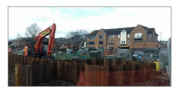
Sheet pile wall in allotments (before cladding). The square piling separate to the wall is for installation of the pumping station.
