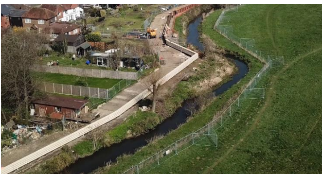
Flood wall upstream of bridge
