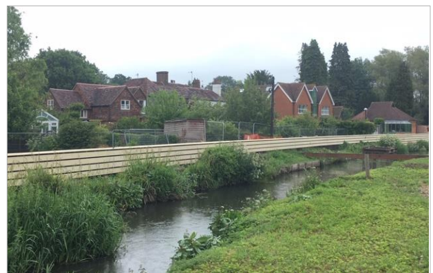
Flood wall completed downstream of bridge
