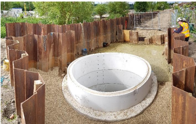
Pumping station construction in Catteshall Road Allotments
