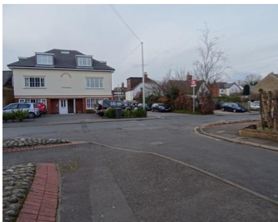
Lack of adequate crossing or street lighting at Farncombe Station
