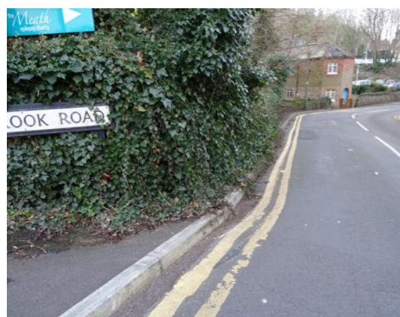
Footway submerged under vegetation
