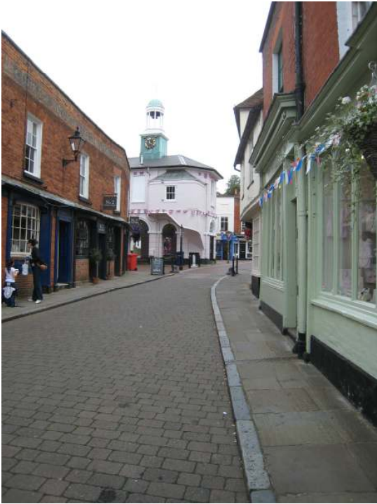
Church Street leading to the Pepperpot showing paving and York stone paving slabs
