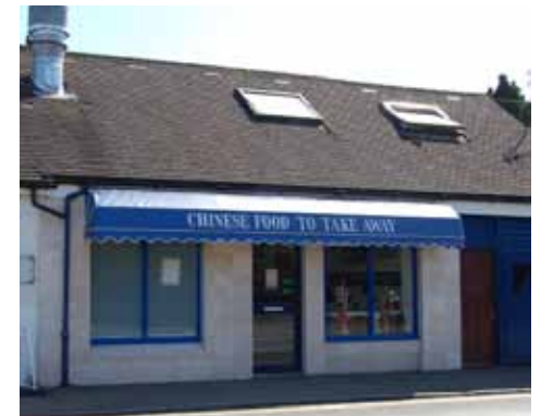
Figure 9. Ewhurst Road, Cranleigh: An example of marble shopfront which is not considered best practice.
