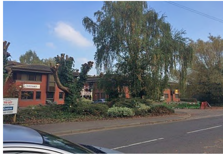
(2) Commercial Offices some of which have been made into flats
