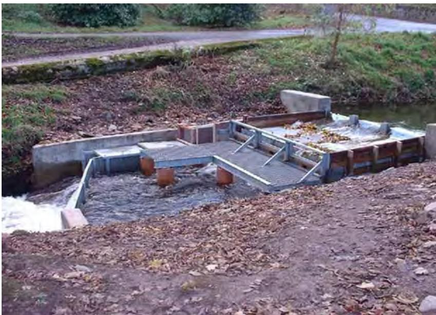
**Figure A10.3 Fish trap (by kind permission of the Tweed Foundation)**
