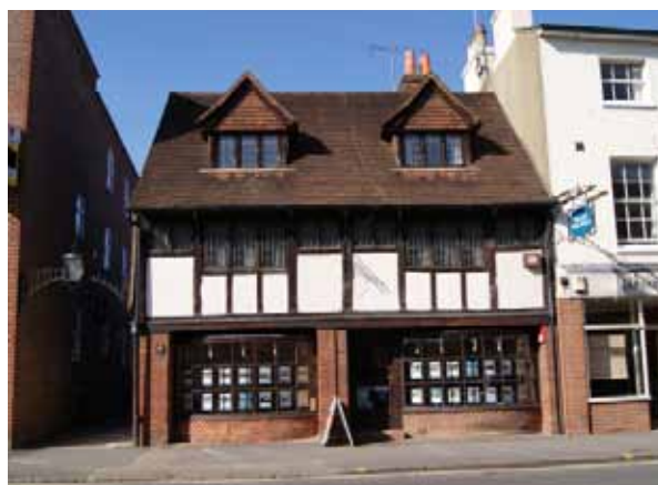
Figure 8. West Street, Farnham: The use of a brick for the stall riser respects the character of the building. The stall riser is proportionate to the building and elevates the window to eye level.
