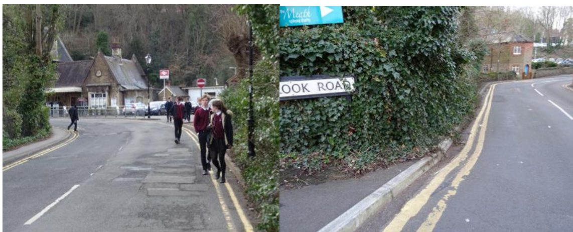
Lack of pavement on the station side of the main route into Godalming Town Centre
