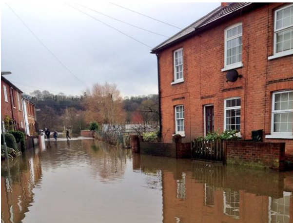
Catteshall Bridge Road flooding Dec 2013
