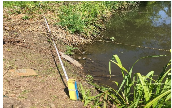
Marking the sheet pile alignment on site
