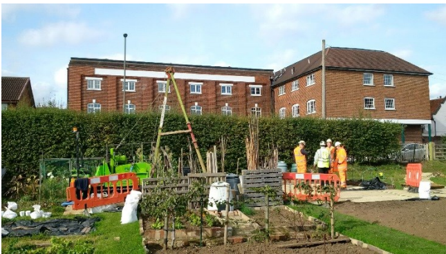
Ground investigation works in the allotments
