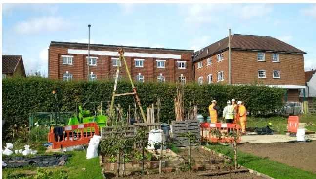
Ground investigation works in the allotments
