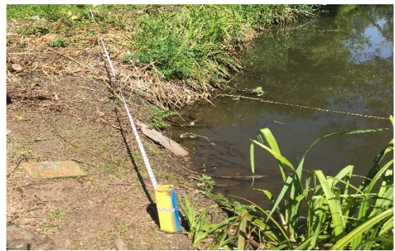
Marking the sheet pile alignment on site
