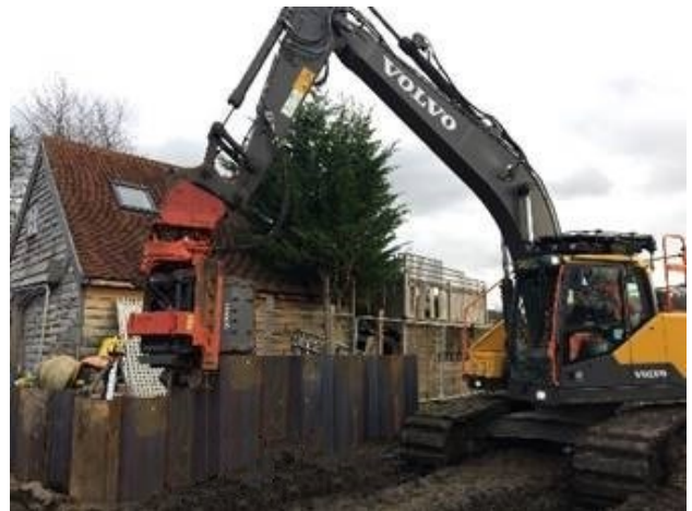
Installing the sheet pile wall at Lammas Cottages
