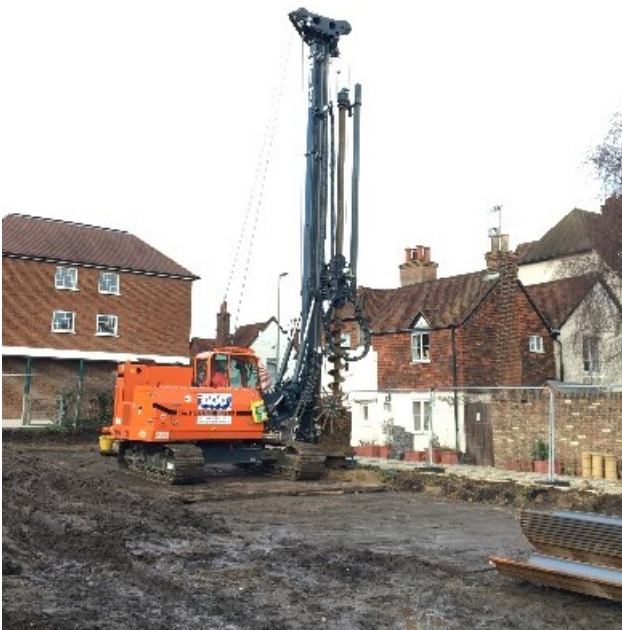
Auger working at Lammas Cottages
