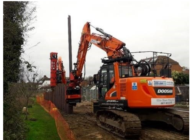
Sheet piling works in allotments
