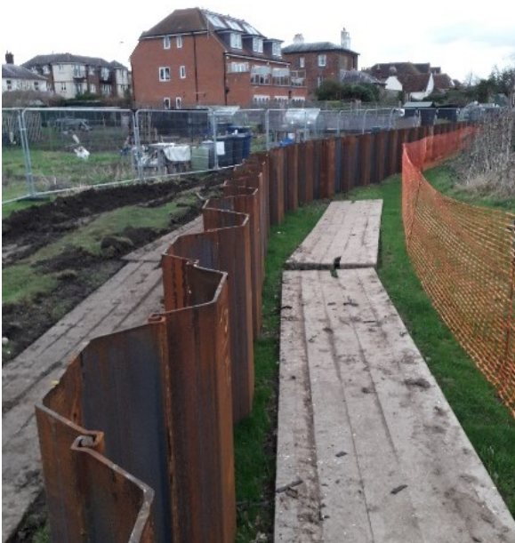
Finished section of sheet pile wall (before cladding)
