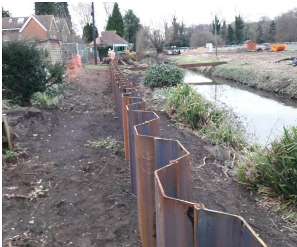
Finished section of sheet pile wall (before cladding)
