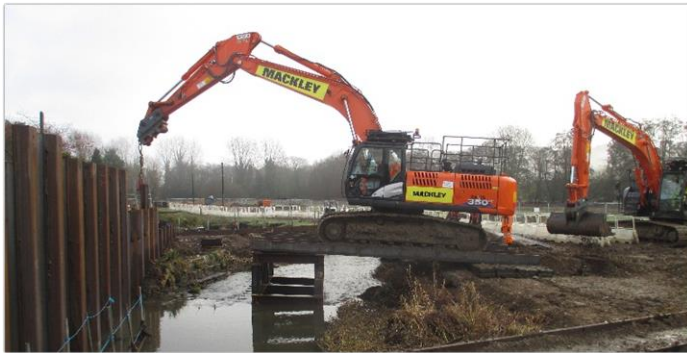
Sheet piling downstream of bridge (Feb 2019)
