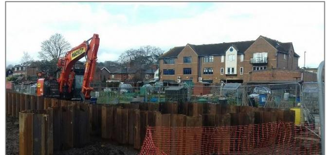
Sheet pile wall in allotments (before cladding). The square piling separate to the wall is for installation of the pumping station.
