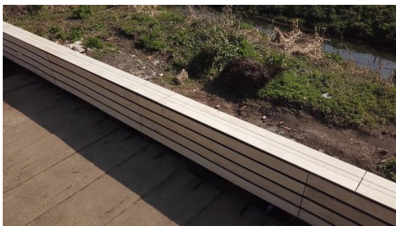
Section of completed flood wall with cladding
