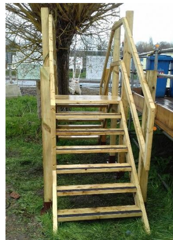
Steps example constructed in front of the site office
