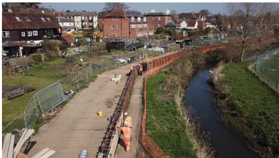
Sheet pile wall with cladding in progress
