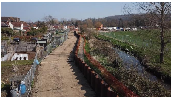
Sheet pile wall awaiting cladding
